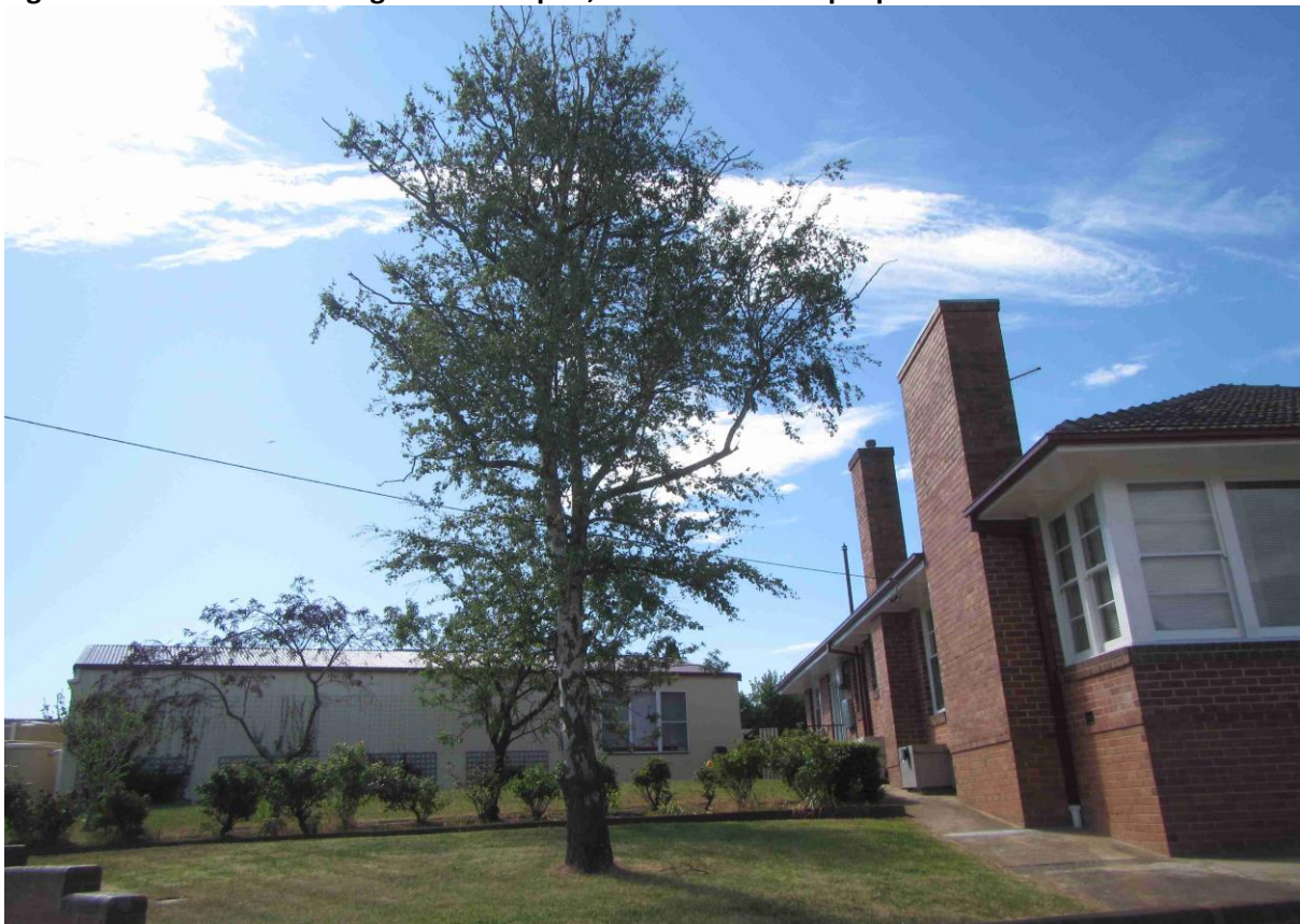
Figure 11 Shows Tree 5 within the front landscape setback to be removed.
